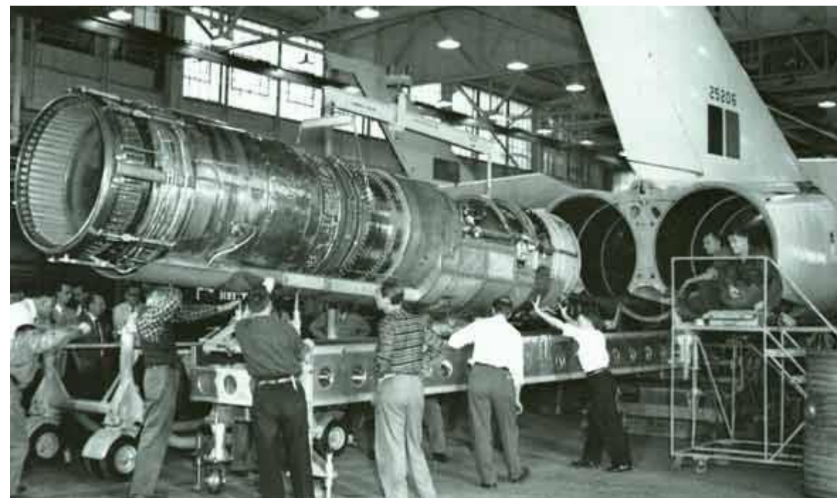
Iroquois being Fitted on RL-206: the only Mk II Arrow ever built
